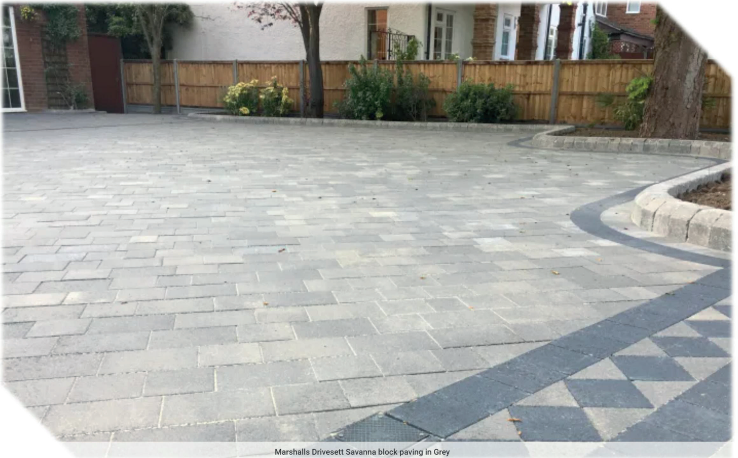
Marshalls Drivesett Savanna block paving in Grey
